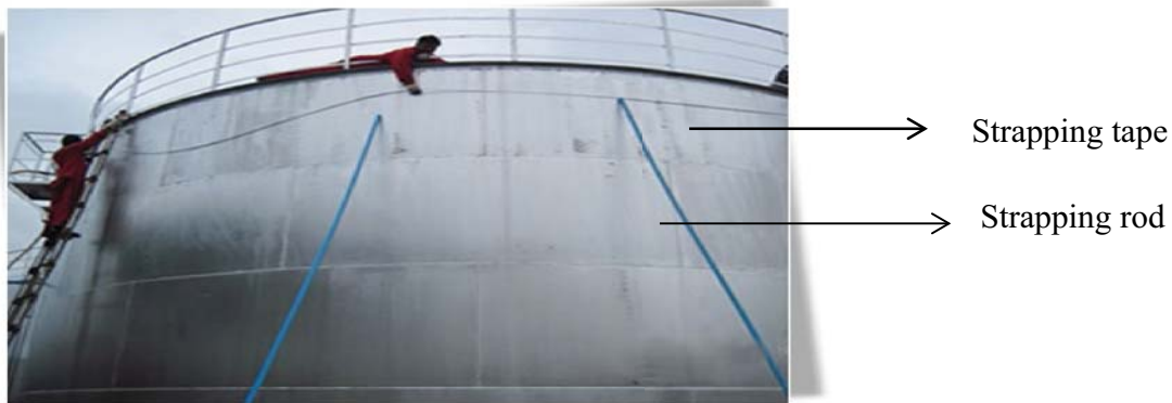
Figure 3: Strapping of tank shell
