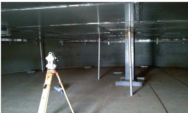
Figure 4: Bottom survey with leveling instrument
